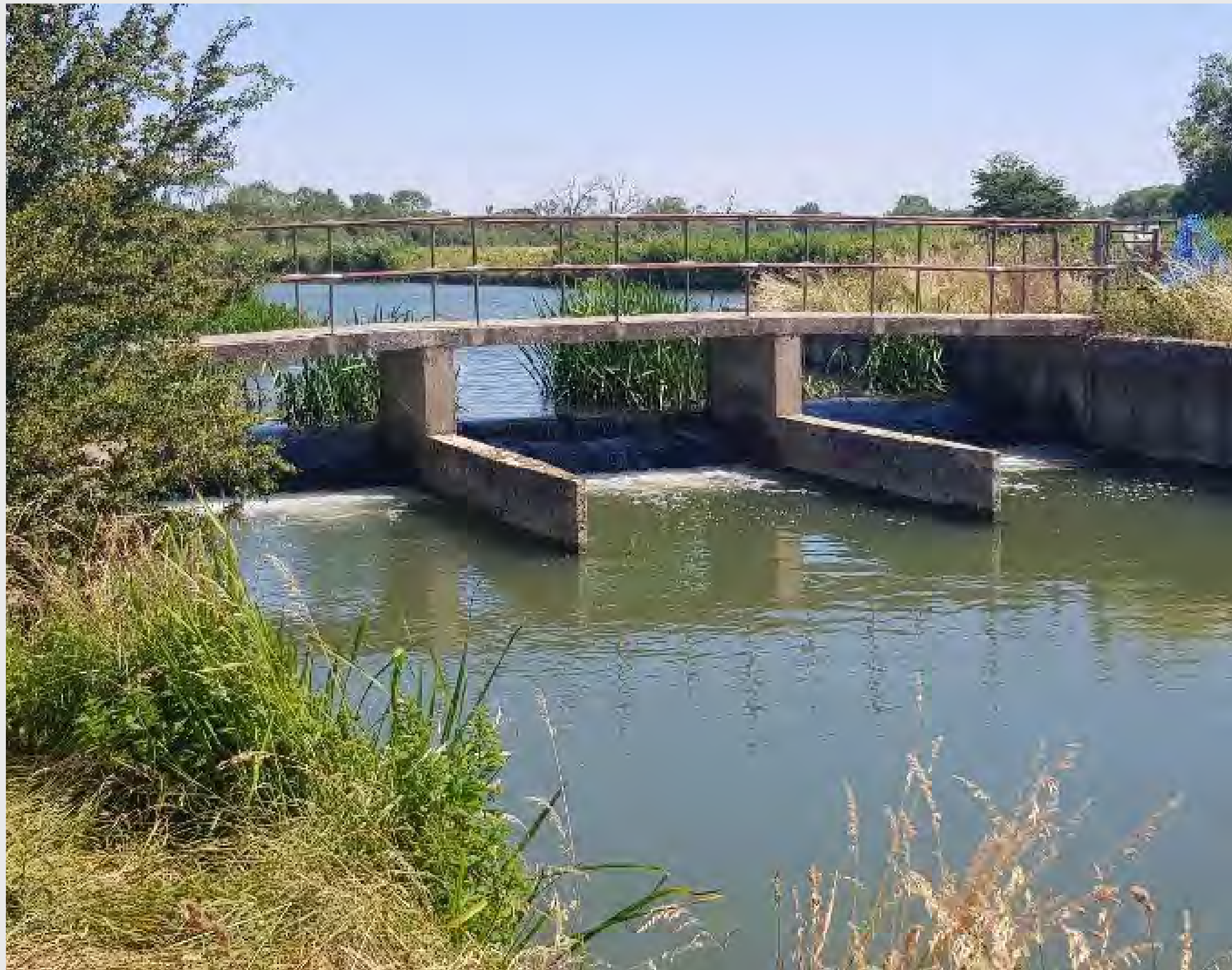
↑ Seacourt Stream Offtake from River Thames – Barrier to Fish Movement
